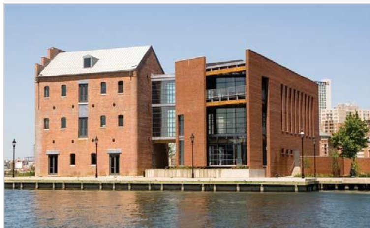
Figure 1 Reused brick is combined with New Brick in this extended commercial building.
